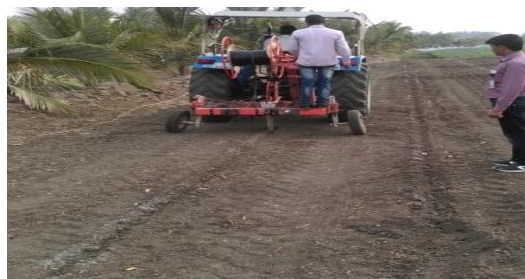
Sub surface drip installation
